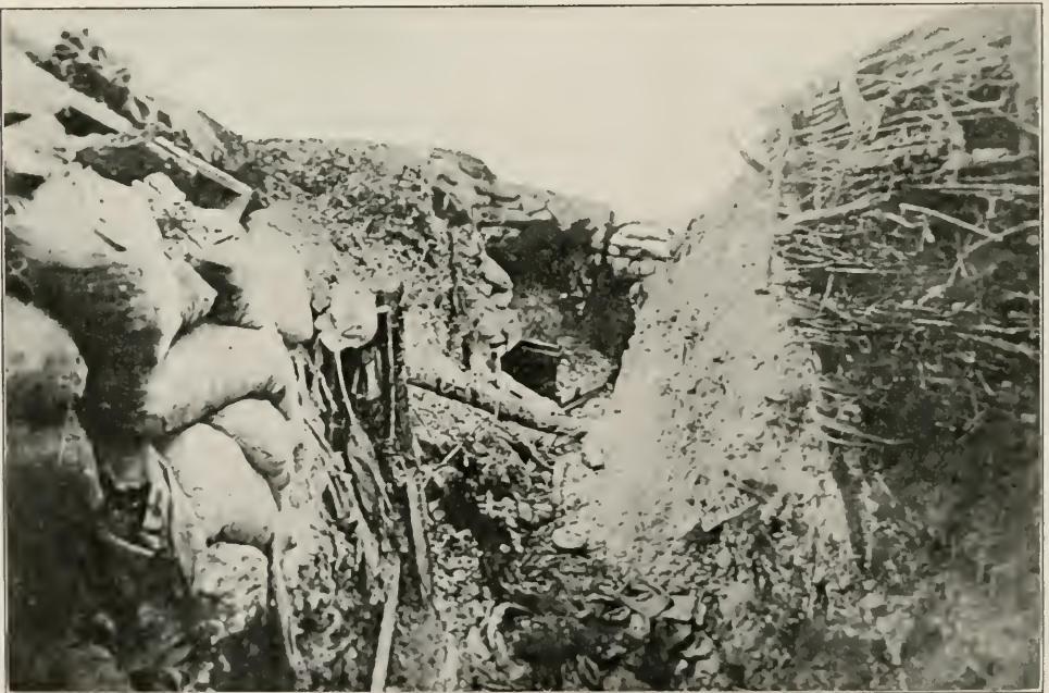
Partly Demolished German Trench
